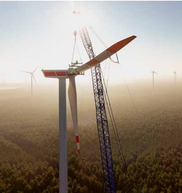
Quelle | Source: eno energy
