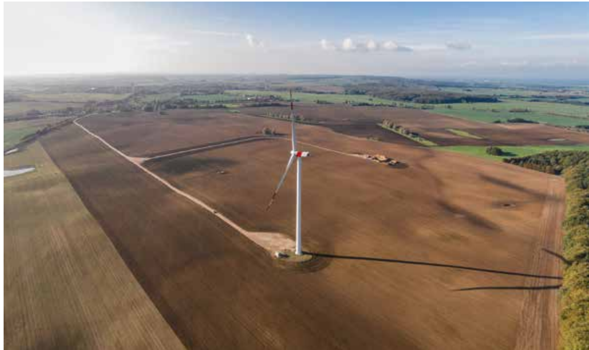
Quelle | Source: eno energy
